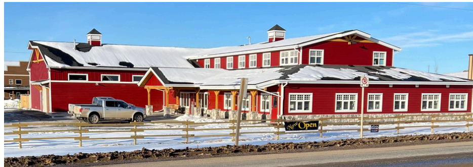
View of the new clinic, from Highway 7.
